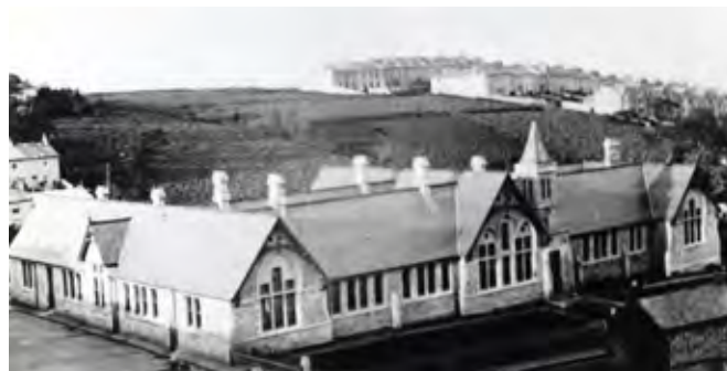
The completed Stennack board school viewed from the south. The left and right wings were for boys and girls, separated as was the custom at the time, while the centre was for infants.
