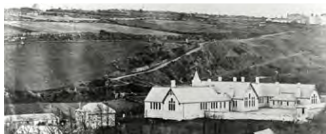
The Stennack board school soon after completion, seen from the north. The dumps of the old Trenwith mine and the long ropewalk near the top are visible on the opposite side of the valley. The headmaster's house is on the left. This was never used by the headmaster and was later turned into classrooms as pupil numbers at the school increased.
