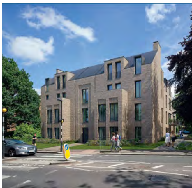
The new almshouses being built at Queen's Road
